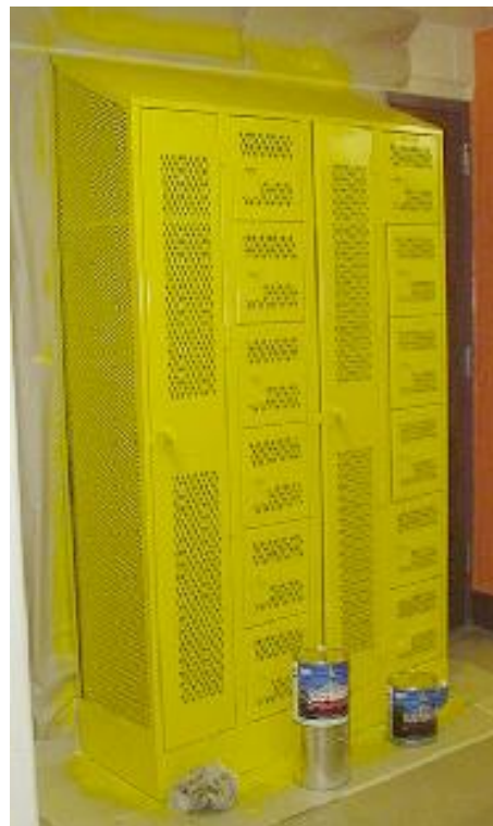
Electrostatic painting in Engelmann Hall.
