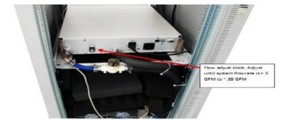
Figure 12: Flow adjustment knob
