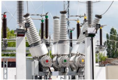
SF<sub>6</sub> gas-insulated switchgear at an outdoor substation.
